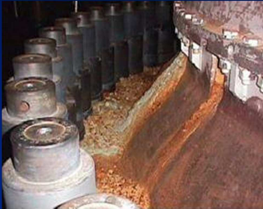
Rod Rusty Boric Acid Deposits on Vessel Flange (12RFO)
